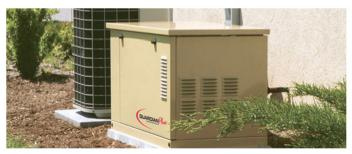
conditioning unit. The generator system will automatically start and transfer loads on a power outage. When utility power returns, the generator system will automatically shut down.
